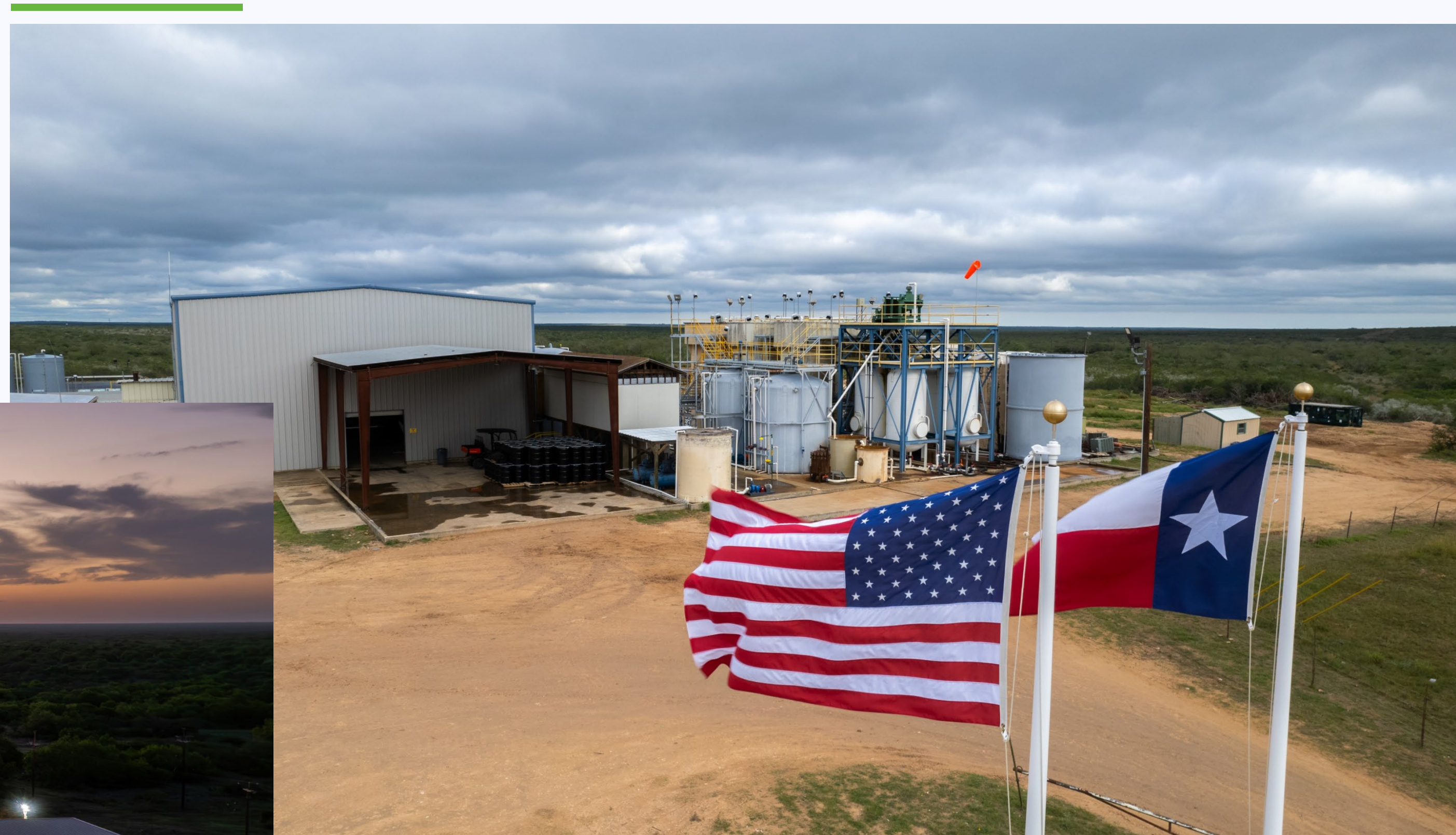
Rosita ISR Uranium Central Processing Plant
