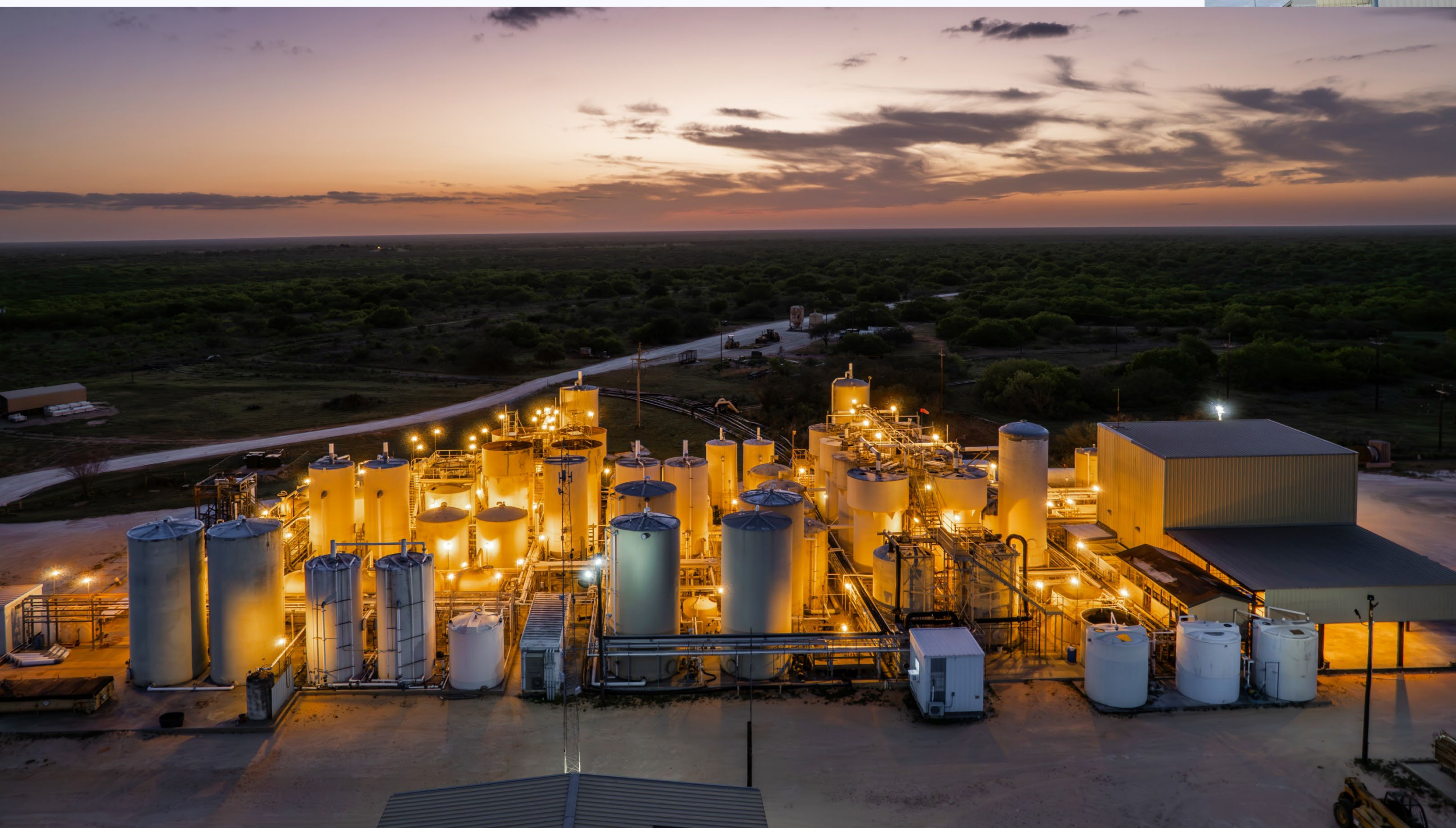
Alta Mesa ISR Uranium Central Processing Plant
