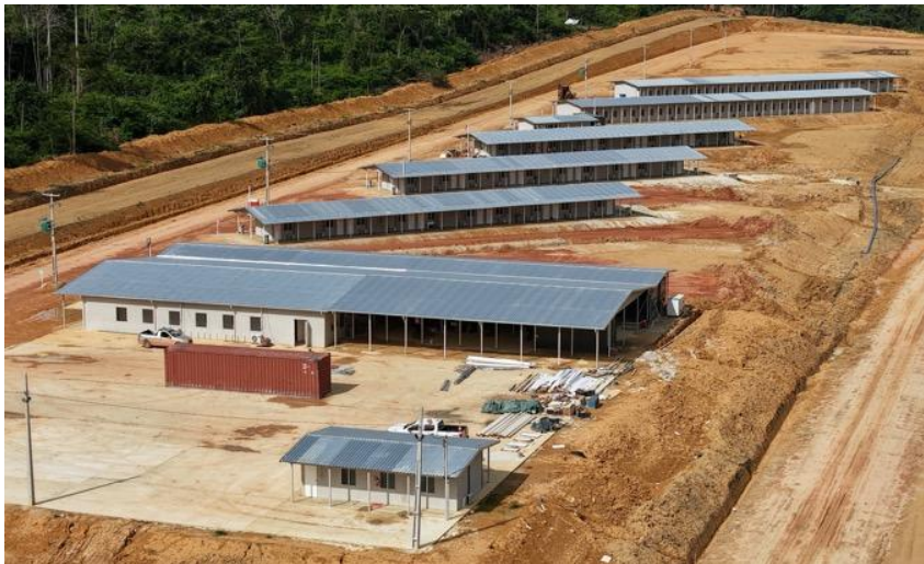
Mine camp for 160 people completed on schedule
