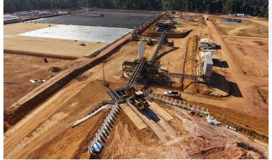
Construction activity in ROM / dry circuit area
