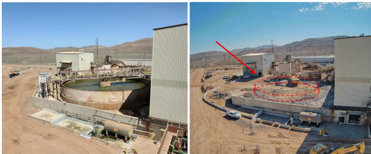
Figure 2: Demolition of the existing CIL tanks in preparation for new CIL tanks as part of the Lone Tree Plant refurbishment.
