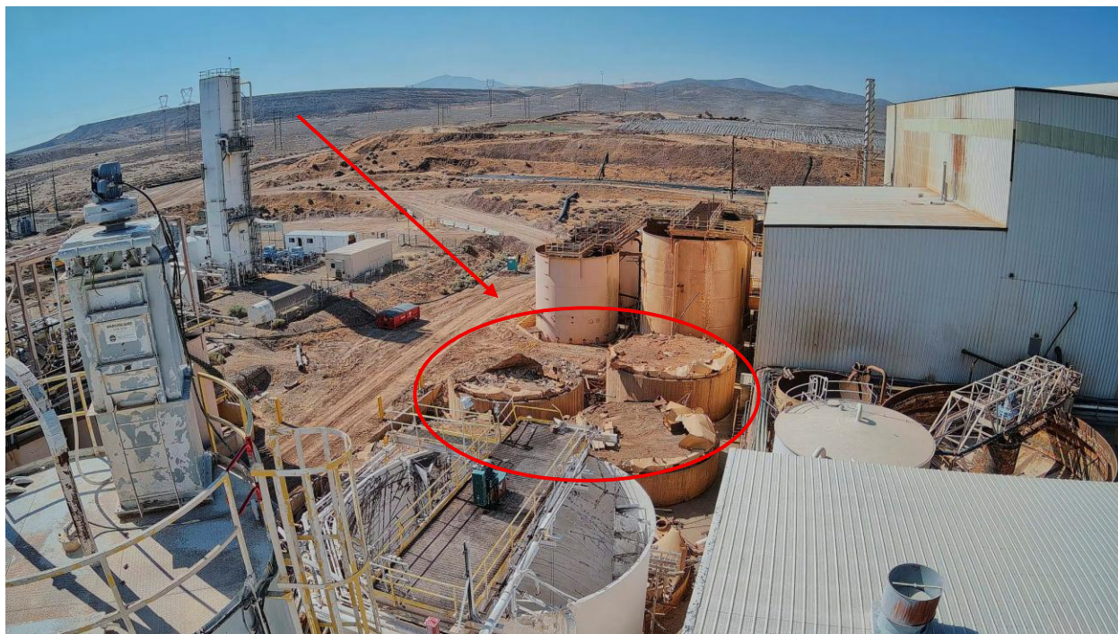
Figure 2: Demolition of the existing CIL tanks in preparation for new CIL tanks as part of the Lone Tree Plant refurbishment.
