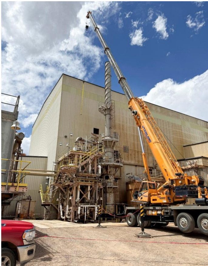
Figure 4: Demolition of the autoclave off-gas system in preparation for the installation of a new mercury capture system.
